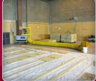
With a 600V service running directly into this studio space this 40 kW furnace was a perfect fit. The safe, dry heat ensured that construction of the set pieces was kept on schedule.
