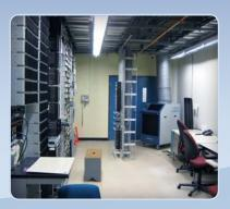
This Telco hub required temporary cooling while the building system was being upgraded. Heat was vented through exhaust air ducts that allowed direct flow out of the building.
