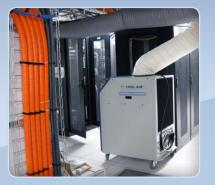
These units have a built-in condensate tank as well as an onboard condensate pump that provides flexibility when it comes to setting these units up.
