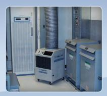
This electrical transformer space benefited from portable air conditioning units when the dedicated cooling failed.
