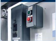
Having a push button control, simply select the green button for full on cooling or push the red button and the unit immediately shuts off.
