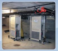
These two units provided 8 tons of temporary cooling to this electrical vault. The vault required cooling in order to be energized by Hydro prior to the dedicated cooling equipment being in place and functional.
