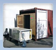
These temporary dimmer shacks are used to store lighting control mechanisms for the movie industry. They build up a tremendous amount of heat and require cooling to maintain operation. These 4 ton units are ideal for this application.
