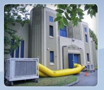
This air cooled package was the perfect fit for this film location. A large amount of cooling was needed from this 25 ton unit to handle the entire building and this 3 ton was ideal for spot cooling cast and crew.
