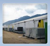
Special events often require large amounts of cooling. These 25 ton units were installed to keep staff and patrons comfortable, even with the hot summer
