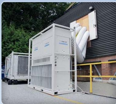
With limited floor space in most telecom rooms, our 15 ton unit was the perfect fit for this temporary application. Able to sit outdoors and duct the Cool Air into the building, optimal temperatures were maintained with minimal disturbance.
