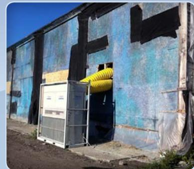
Film locations often require units that can be kept out of the way. This 15 ton unit was situated outside the space being used. The crew were able to operate the unit from inside using our push-button remote. The electric heating capabilities of these units allow for easy change over from cooling to heating.
