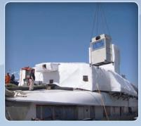
While in drydock, the dedicated chiller on this yacht was pulled for rebuilding. This unit kept the temperature below deck comfortable for the crew.
