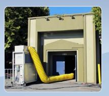
This 10 ton unit handled the summer heat and kept the inside of this film location comfortable.
