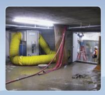
Prior to being energized by the electrical utility, this vault needed to be cooled by this 10 ton unit. Once the dedicated unit was brought online, we simply rolled ours out of the underground parking area.
