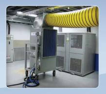
The dedicated cooling unit in this electrical vault failed in the height of summer. Quick response with this 8 ton unit meant the proper operating temperature was restored and the industrial facility was operating normally within hours.
