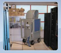
Fitted with the alternate 90° plenum, this 5 ton directed its full cooling strength at the server cabinet.
