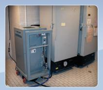
The freezers in this lab outstripped the capacity of the dedicated unit. With the addition of this supplemental unit, acceptable temperatures were restored.
