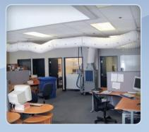
A localized cooling problem in this office area was solved by installing this water cooled unit. Perforated duct was utilized for maximum coverage.
