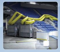
This stadium event required a large amount of cooling equipment to run continuously. By positioning the units away from the stage and running flex duct through the back of house area, we were able to deliver air to the event all day long.
