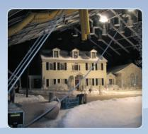
This large temporary structure was built around this full sized house. The structure allowed for night scenes to be filmed during the day. Filming took place during July and August, meaning that the heat inside the structure needed to be managed.
