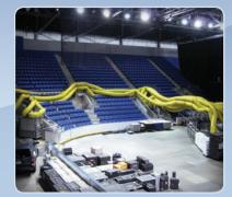
The requirements of this event dictated that the units be located a distance from the stage. Our back of house location meant that, while long, the duct runs needed to remain effective.
