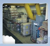
This warehouse was unbearably hot during the summer months. Installing a dedicated system was not cost effective so this 20 ton unit was brought in for four months. It kept the facility nicely cooled so that the staff could hide in the racking and sleep.
