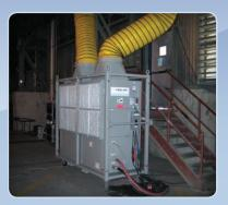
This industrial facility had its dedicated cooling system down for maintenance. Problems with parts meant the week that the project was planned to take, turned into a month. This 20 ton handled the heat more effectively than the building system, and when the job ended, we simply rolled the gear out the door.
