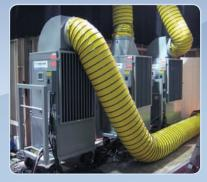
This movie set required a large amount of cooling but site constraints dictated smaller mobile units that could deliver precision cooling to specific areas. These 10 tons exceeded expectations.
