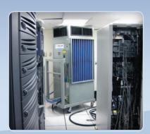
Server room cooling applications are an ideal fit for this unit. Outfitted with hard nylon tires and a low profile plenum, these units slip into any server room.
