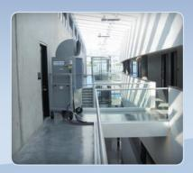
This atrium approached meltdown when the ventilation system quit working, This 10 ton unit restored reasonable air temperatures and the classrooms surrounding this space were not met with a wall of heat when the doors opened.
