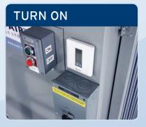
Easy switching between thermostat controls and on/off push button control makes operating this unit a snap.
