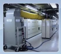
Equally adept at precision cooling, this 10 ton unit was called upon to provide emergency cooling to this electrical vault. The perforated industrial duct was used to deliver air directly to the electrical cabinets.
