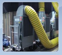
This movie set required a large amount of cooling. Site constraints dictated smaller mobile units that could deliver precision cooling to specific areas. These 10 ton units exceeded expectations.
