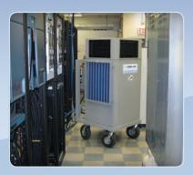
These 5 ton units are the backbone of our water cooled fleet. They are the "go to" machines when server room cooling problems surface.
