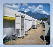
Temporary structures like these are an ideal application for these vertical 4 ton units. These tents required cooling to ensure that staff and patrons were able to function properly in extremely warm conditions.
