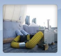
Flexible ducting was connected to fittings on this inflatable structure. Warm air was delivered inside to make sure guests were comfortable in the height of winter. Heaters of Olympic proportions are what Cool Air is all about.
