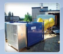
Most commercial buildings will have the load capacity to handle rooftop placement of this lightweight unit. With the ability to be connected to the building DDC system, remote activation and control is as simple as can be.
