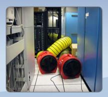
When a large amount of ventilation is required but space and power are at a premium, these floor fans are the perfect fit. Able to be ducted, they can bring in clean, filtered air right where it is needed.
