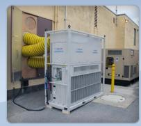
This site needed ventilation and dehumidification which made this air cooled 20 ton unit a perfect fit. Optimal conditions can be met and retained with this easy to use unit.
