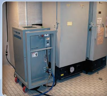
The freezers in this lab outstripped the capacity of the dedicated unit. With the addition of this supplemental unit, acceptable temperatures were restored.
