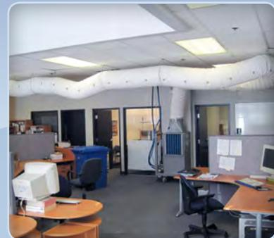
A localized cooling problem in this office area was solved by installing this water cooled unit. Perforated duct was utilized for maximum coverage.
