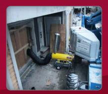
Small scale construction heating projects are a perfect match for this specialized heating unit. Separate combustion air allows for high temperature supply air but with a low humidity level. Dry air enables moisture trapped in construction materials to be released resulting in a drier project.
