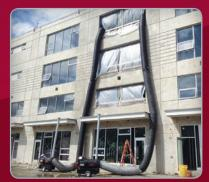
Construction sites with limited power can effectively be heated with these easy to use units. The additional heat was required to control humidity levels when drywall was being installed.
