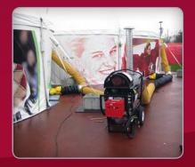
These promotional Olympic tents were kept dry and comfortable because of this gas fired heater. The separate pods of this structure required individual duct runs.
