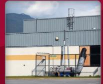
While the dedicated boilers and air handling units were being replaced, these natural gas fired units provided temporary heating for this community centre. All programs and services were kept operational avoiding a costly shutdown.
