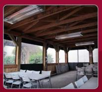
This permanent shelter requires heating during the cooler months. Temporary 6 kW heaters were the perfect fit for this drafty space. Radiant heaters are exceptionally good at providing comfortable conditions where other styles of heating fail.
