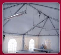
These radiant panels are great for temporary structures such as this tent. Heating the people inside the tent instead of the air ensures that the heat energy is used to maximum effect.
