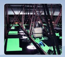
A specialized projector was located in the truss area of this Film Stage so that images could be projected down to the studio floor. The projector generated a lot of heat and if subject to high operating temperatures it would shut off. Our Super Cooler was hoisted into place to pump conditioned air in to the cabinet and keep it operational. The aluminum frame allowed the Riggers to easily secure this unit in place.
