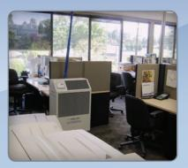
When this building system failed at the peak of a heat wave, four of these 1.5 ton portables were installed and comfort levels were restored. This was an ideal application for a premium portable unit.
