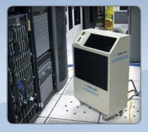
For emergency applications, where the temporary cooling solution has to be running immediately, these plug-in units are the perfect fit.
