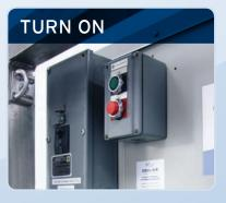
Having a push button control, simply select the green button for full on cooling or push the red button and the unit immediately shuts off.
