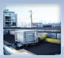
Rooftop placement allows for effortless integration with your existing duct system. Remote thermostat ensures that desirable temperatures are maintained.
