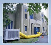
This air cooled package was the perfect fit for this film location. A large amount of cooling was needed from this 25 ton unit to handle the entire building and this 3 ton was ideal for spot cooling cast and crew.
