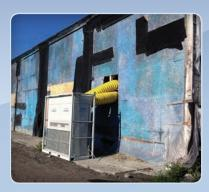
Film locations often require units that can be kept out of the way. This 15 ton unit was situated outside the space being used. The crew were able to operate the unit from inside using our push-button remote. The electric heating capabilities of these units allow for easy change over from cooling to heating.
