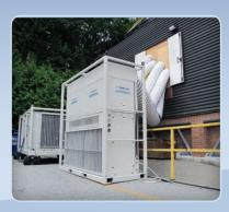
With limited floor space In most telecom rooms, our 15 ton unit was the perfect fit for this temporary application. Able to sit outdoors and duct the Cool Air into the building, optimal temperatures were maintained with minimal disturbance.
